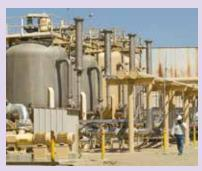
softening system ready for the once through steam generator, followed by media filtration, ion exchange softening, and a double pass reverse osmosis system.
